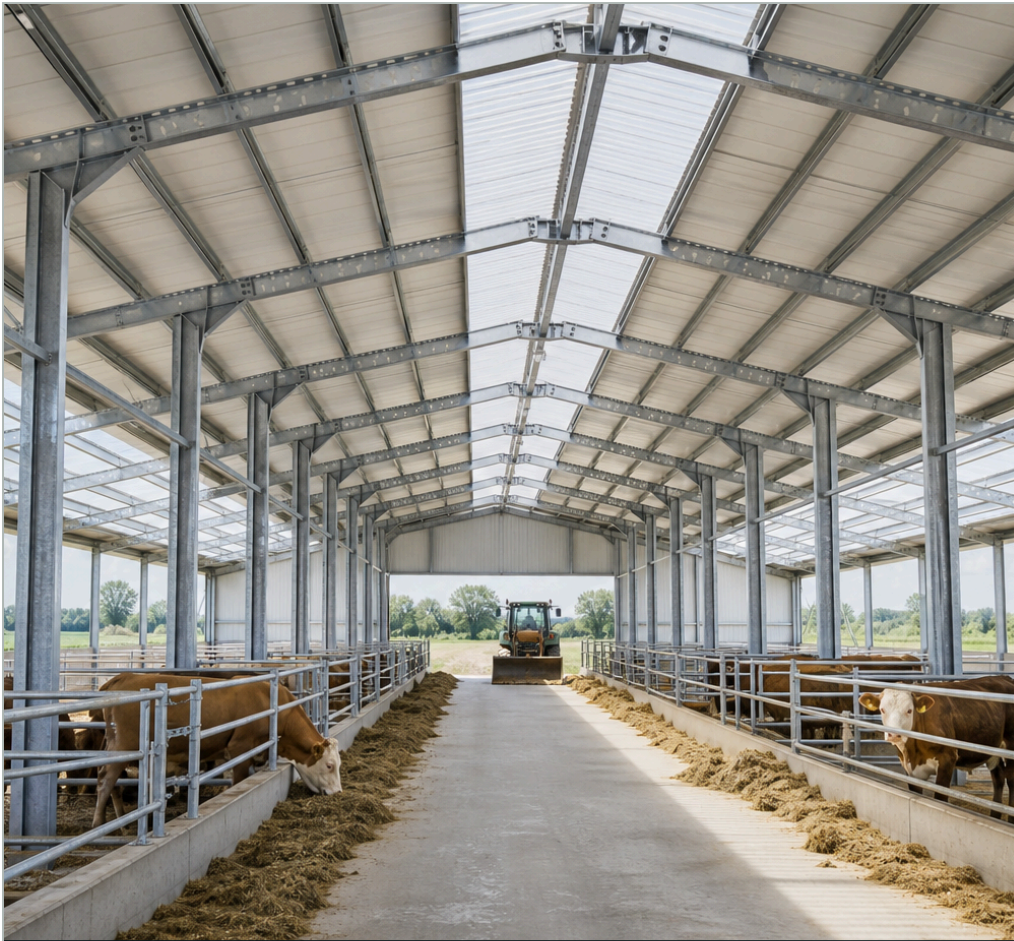
Natural ventilation, generous access and an operation-specific interior layout.
